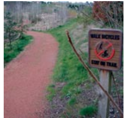
The loose surface of this path and its narrow width make it unsuitable for bicycles. Clear signage indicates the appropriate use. Photo credit: Institute of Transportation Engineers Pedestrian and Bicycle Council
