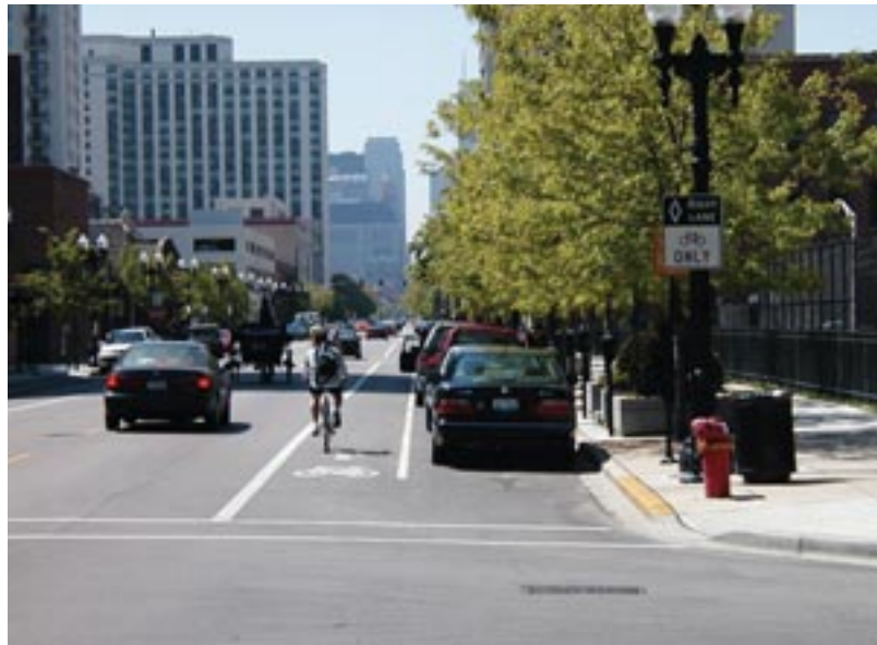
A major consideration when planning bike lanes is the interface between bikes and parked cars. In this photo, the wider bike lane enables the bicyclist to pass the open car door with minimal conflict with moving vehicles to the bicyclist's left. Photo credit: Norm Cox.
