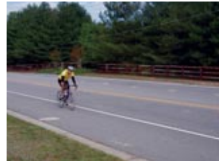
This paved shoulder provides sufficient space for enjoyable and safe cycling on rural roads. Photo credit: Mark Fenton.
